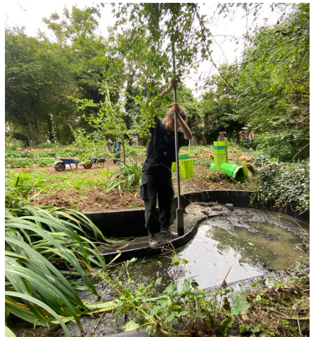
Piercing the module liner to drain water. Photo: Michael Smythe.
