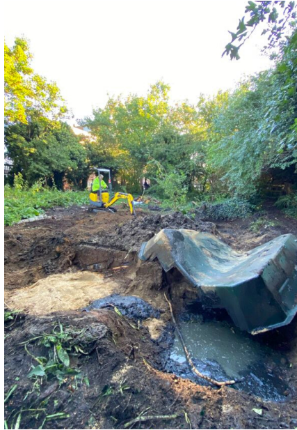
Digging and removing earth. Photo: Michael Smythe.
