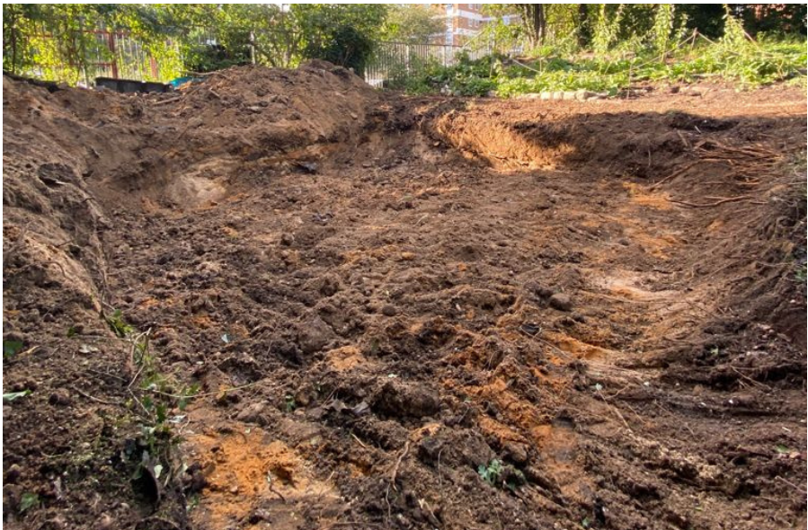
The excavated wetland site. Photo: Michael Smythe.
